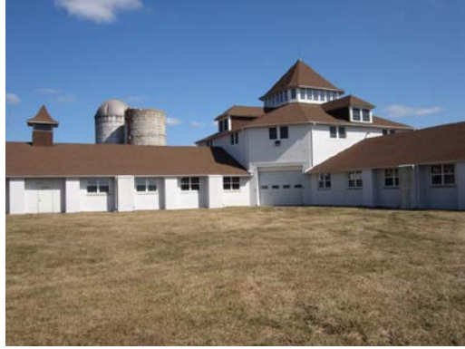
Dairy barn at Norristown Farm Park
